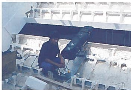
A Golden Scan, positioned above a lower window ledge in the shopping mall's atrium.
